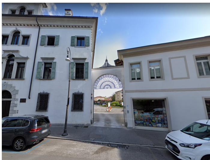
Street view of the main entrance (via Treppo 5/b)
